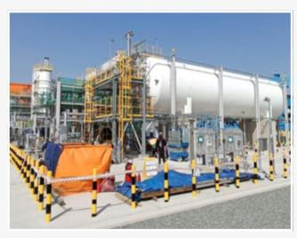
Photos supplied by INOXCVA show four 311,000L liquid hydrogen tanks manufactured by INOXCVA in India for one of the largest prestigious projects for liquid hydrogen in South Korea. The liquid hydrogen is stored in vessels and is used for charging stations nationwide for buses, trucks and trams — with hydrogen as the ultimate clean fuel.
